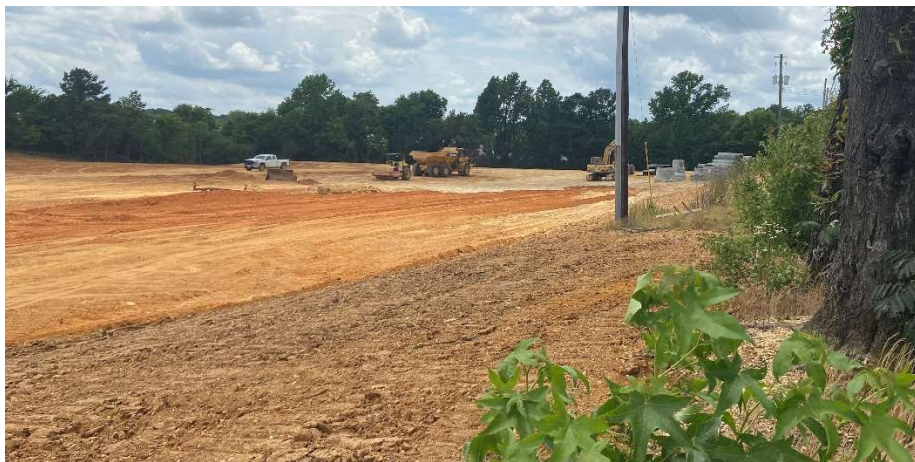
View of the New Facility Location Looking West
