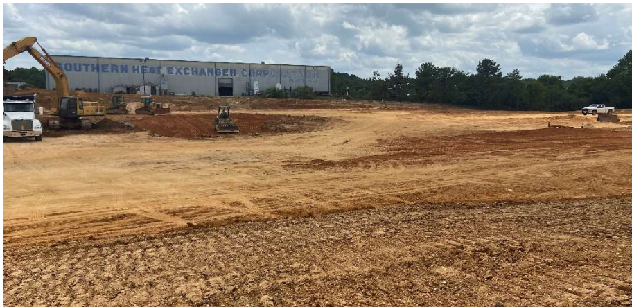
View of the New Facility Location Looking South
