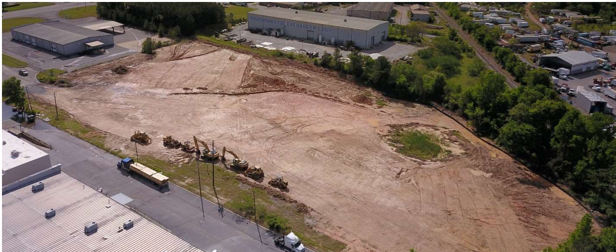
View of the New Facility Location Looking South
